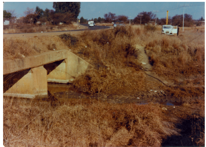
Auguring near the old box culvert north of town.
