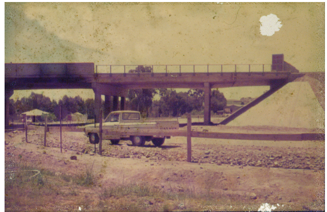
Clocolan “road-over-rail-and road” Overpass project in the winter of 1975, shortly as after its completion – (but see the black smoke marks!)
