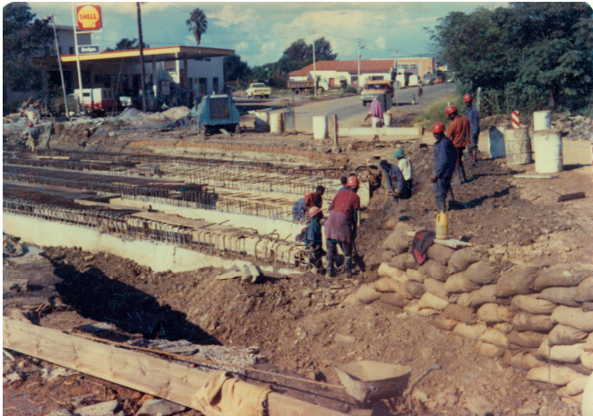
At this site on P 2-2, we did not even have a proper detour! This photo looks east, at the downtown.
