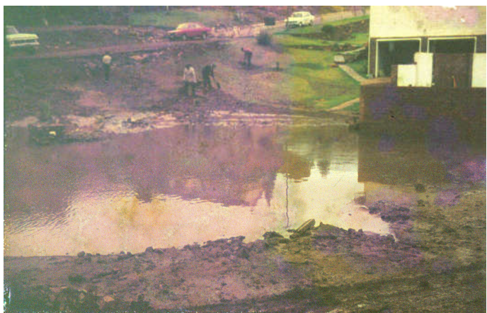
House almost flooded due to blocked stormsewer in higher-up block. Photo taken toward the south.
