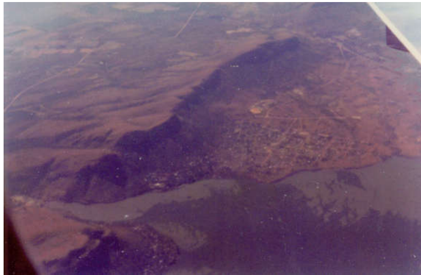
Dam wall Kosmos Schoemansville
