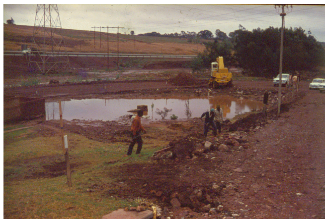
But it was a major storm event. Pond between the "link road" and the highway to Germiston at rear.
