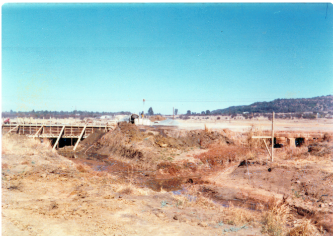
New structure (left) and old box culvert (right) on the road to Lindleyspoort. This photo looks east.
