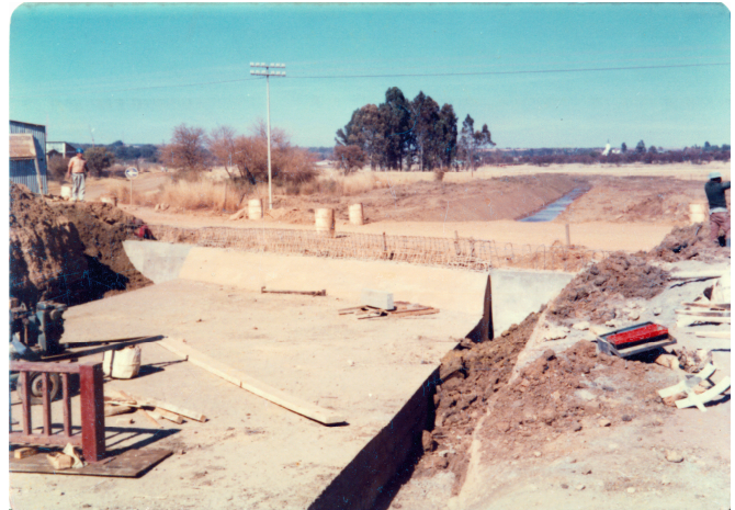
But on P 124-1, north of Swartruggens we had one. This photo looks east, toward the completed ditch.
