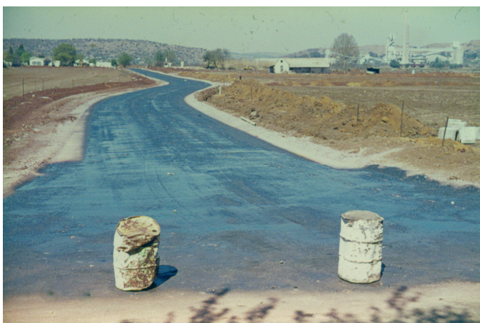
Prime coated Adriaan Street, from Franzina Street. School site is at right, as well as PPC factory.
