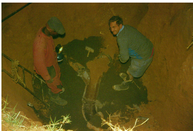
Sanitary sewer connection installed at nighttime. A new manhole was to be built at this connection.
