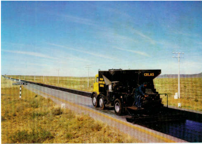
Shown above is the 70 cubic yard Colas Slurry Machine employed on an 81 mile resealing contract for the O.F.S. Roads Department.
