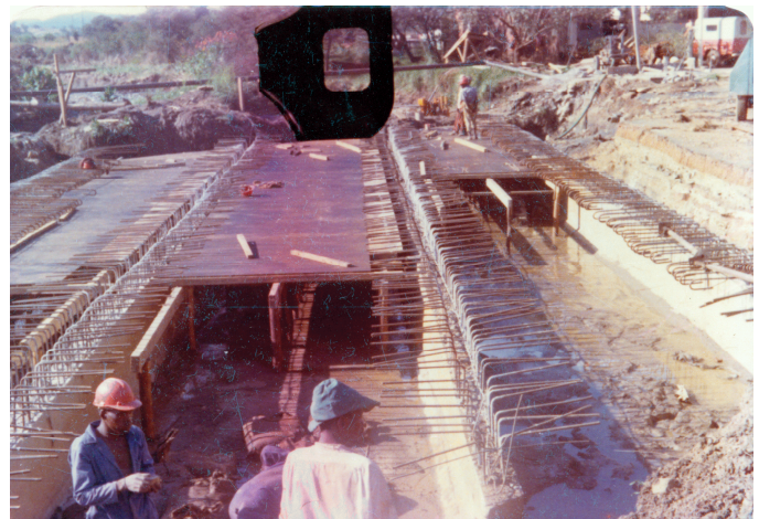
Installation of steel reinforcing for the deck of the 3 x 10' w x 3' h box culvert in Swartruggens.
